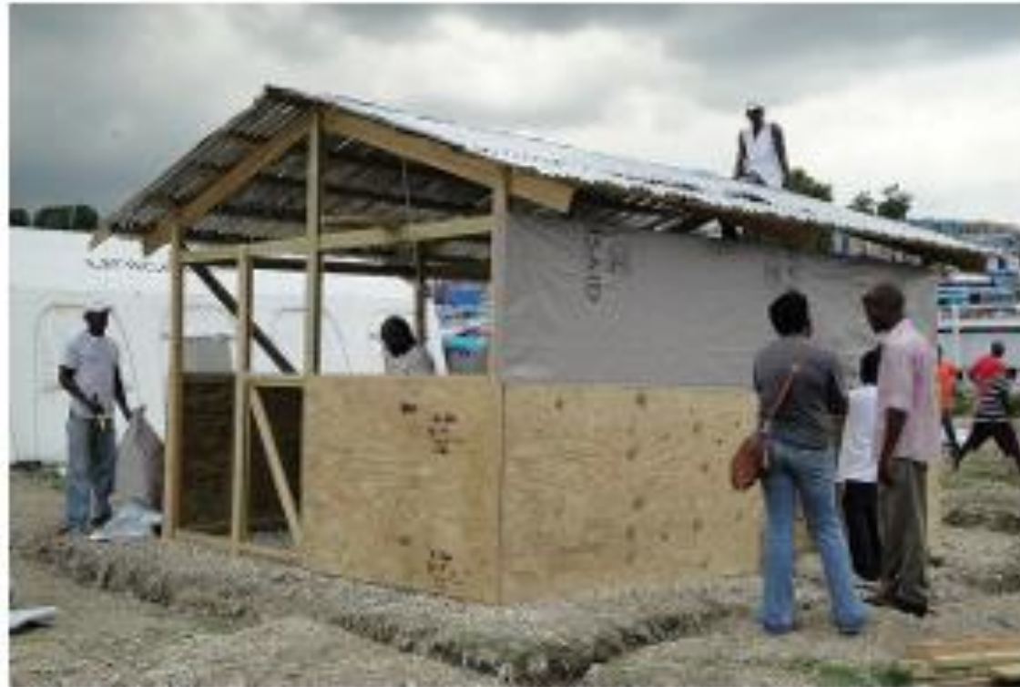
Figure 2 Transitional shelter: See page 14 for more on the transitional shelter concept innovation.
